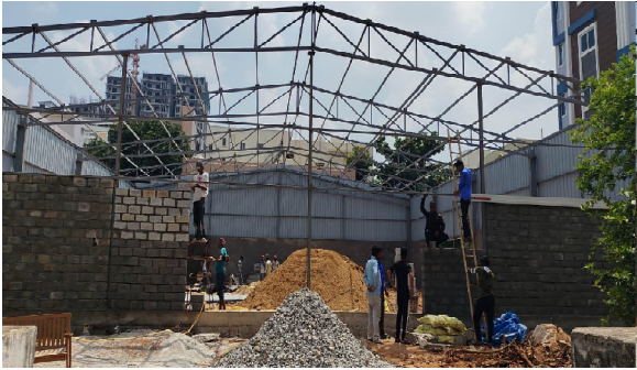
View of the construction of the shed opposite Bethel Sennett School, Maitri Nagar Colony
